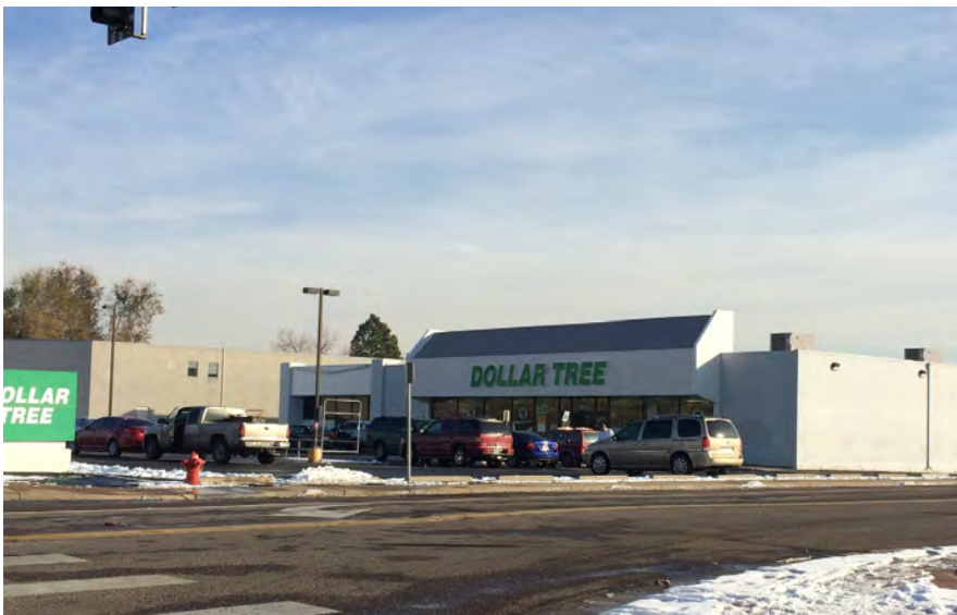
Site Vicinity Retail along West 72nd Avenue
